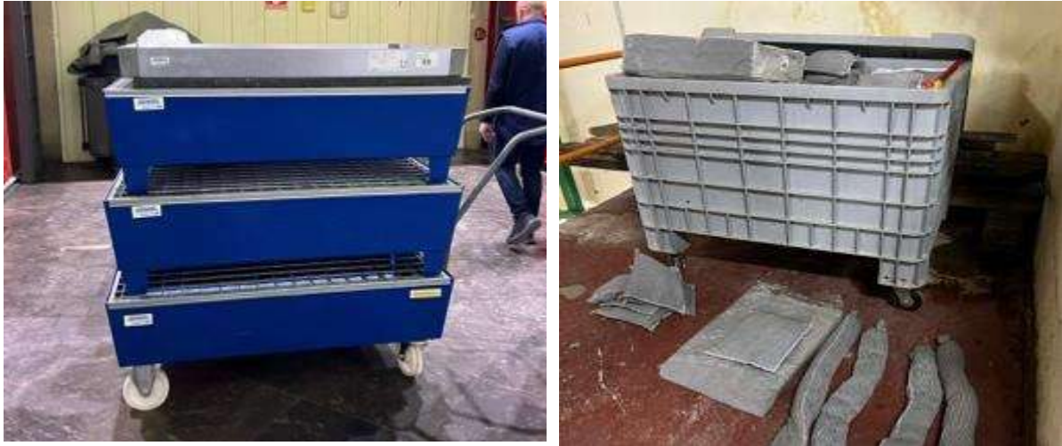
Figure 6-9. Examples of equipment at Jajce II HPP for oils spill prevention
