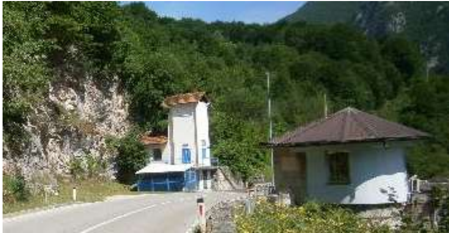
Figure 6-10. Security check point at the Jajce II HPP dam (left)
