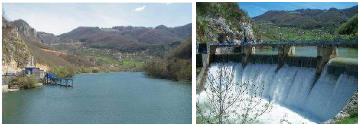
Figure 5-2. HPP Jajce 2- Concrete gravity dam and reservoir (Source: EPHZHB)
