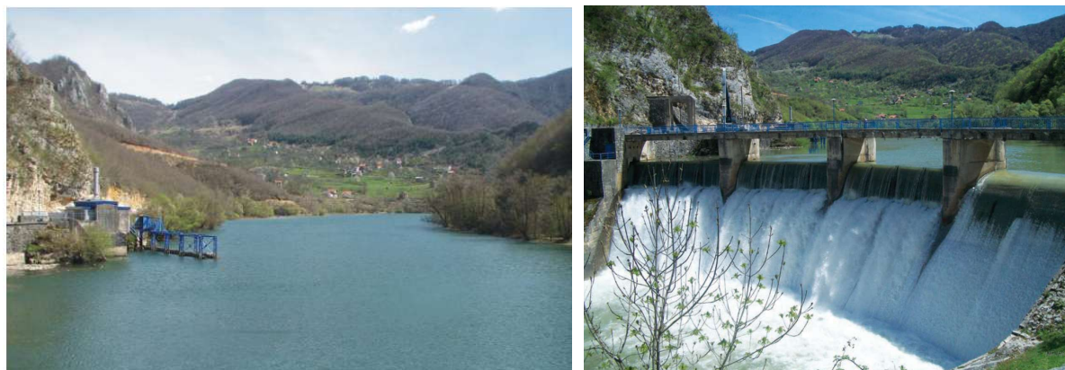
Figure 3-4. HPP Jajce 2 Concrete gravity dam and reservoir (Source: EP HZHB)
